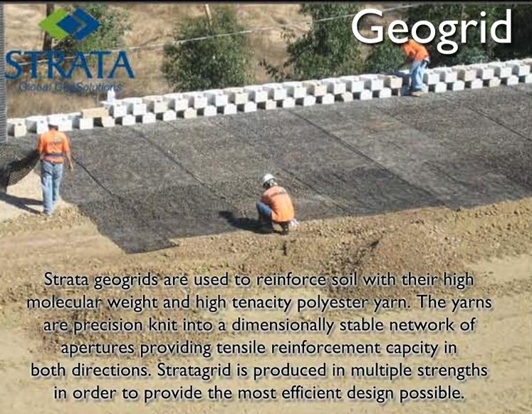
Strata geogrids are used to reinforce soil with their high molecular weight and high tenacity polyester yarn. The yarns are precision knit into a dimensionally stable network of apertures providing tensile reinforcement capacity in both directions. Stratagrid is produced in multiple strengths in order to provide the most efficient design possible.
